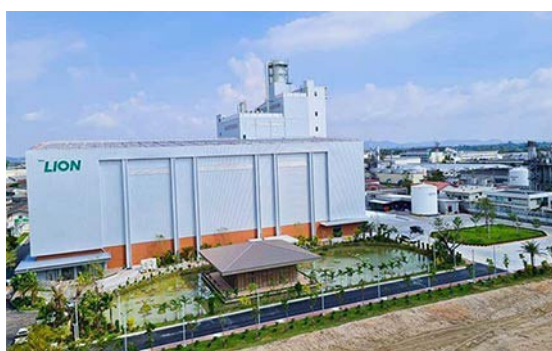
Exterior view of the new drying tower building at LCT
