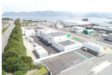
New employee facility building at the Lion Chemical Corporation Oleochemical Production Site (LCCOC)
